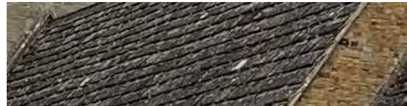
Horsham Stone slate roof
